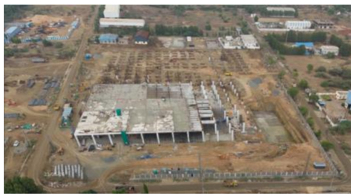
Exhibit 53: Aerial view of the 24-acre PCB-M campus at Nadiupeta, Andhra Pradesh; foundation and structure works underway
